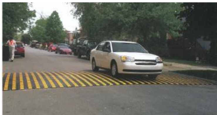
Figure C. Temporary Speed Hump
